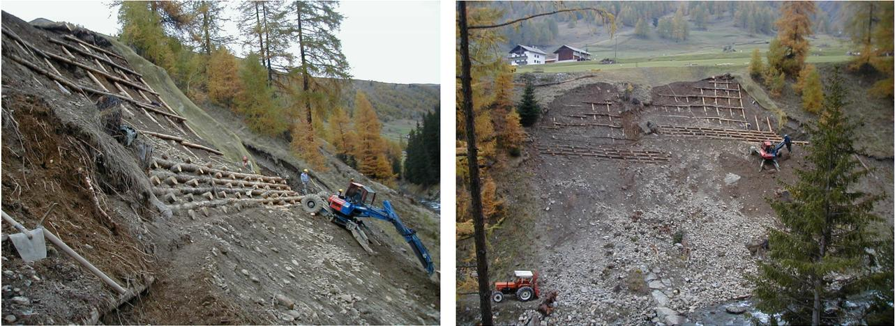
Fig. 7 Construction of a vegetated slope grid based on a vegetated cribwall – Karlinbach 2001
