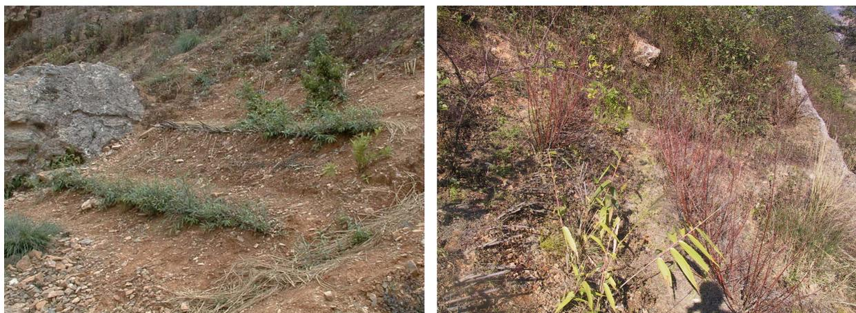
**Fig. 9** The hedge brush layer construction shortly after completion (left)- 2001 and about one year later (right) –2002 in Thankot (Nepal)
