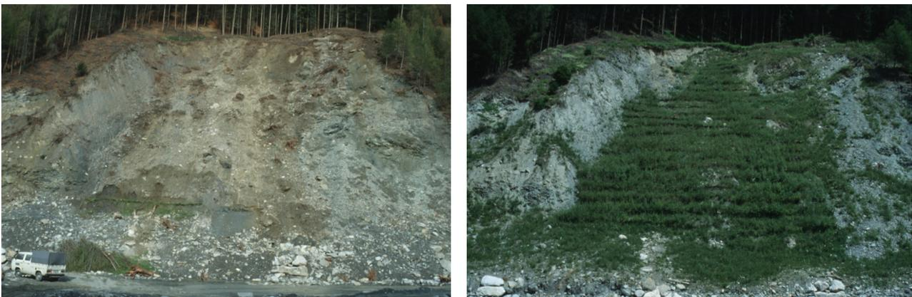
**Fig. 4** Overview of the project area Suldenbach (Italy) beginning with the implementation of hedge brush layers (left)- 1989 and after developing 3 years (right) - 1992
