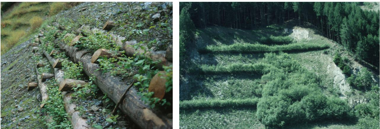
**Fig. 6** A detail of a vegetated cribwall after 6 months (left)–1994 and after 4 years developing (right)-Suldenbach-1998
